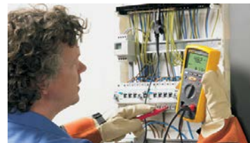
Insulation test at a distribution panel
